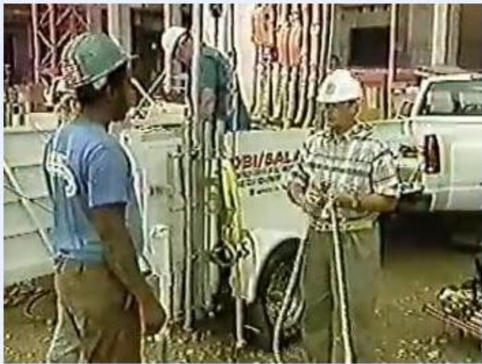
Supervisor in a white hard hat demonstrating rope handling to a group of workers, with safety equipment visible in the background.
