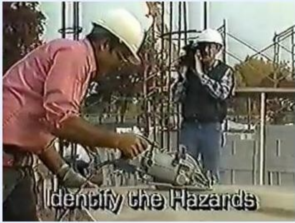
Worker using a power tool while another documents the process; on-screen text reads "Identify the Hazards."
