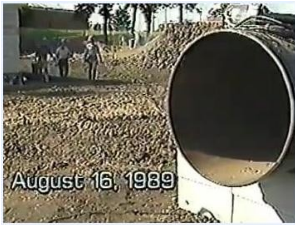
Outdoor construction site showing a large pipe and a job date of August 16, 1989, with three workers visible in the background.
