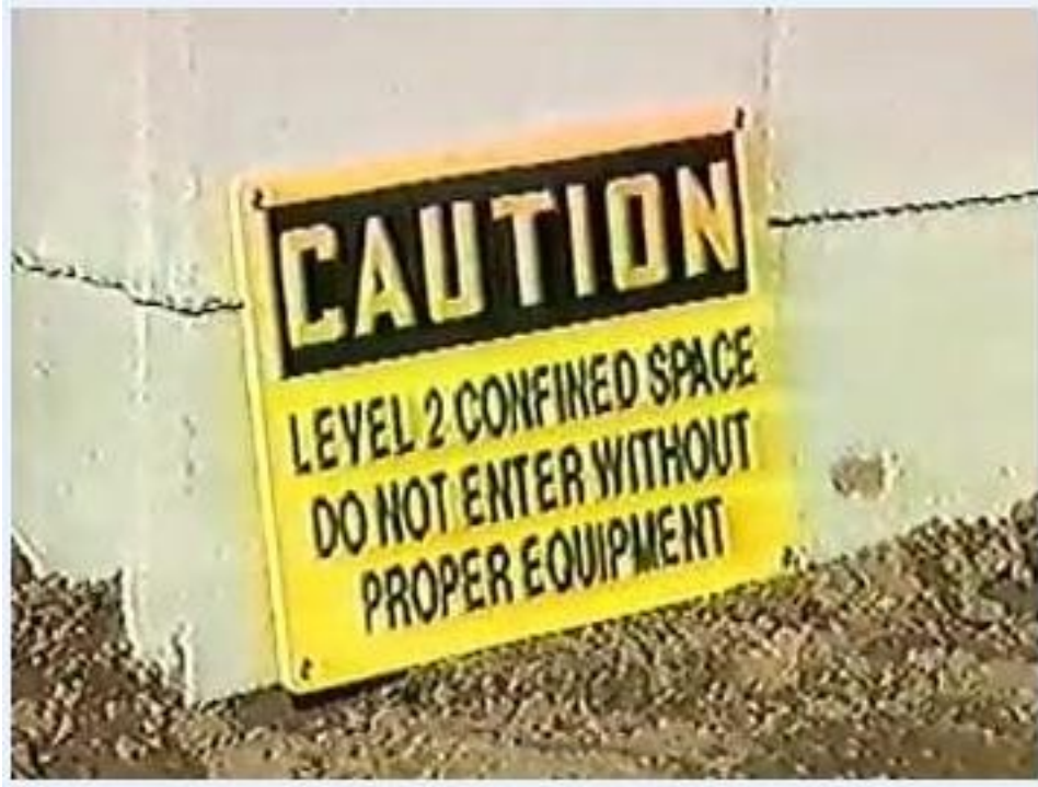
A yellow caution sign reading "LEVEL 2 CONFINED SPACE DO NOT ENTER WITHOUT PROPER EQUIPMENT," posted on a wall at a construction site.
