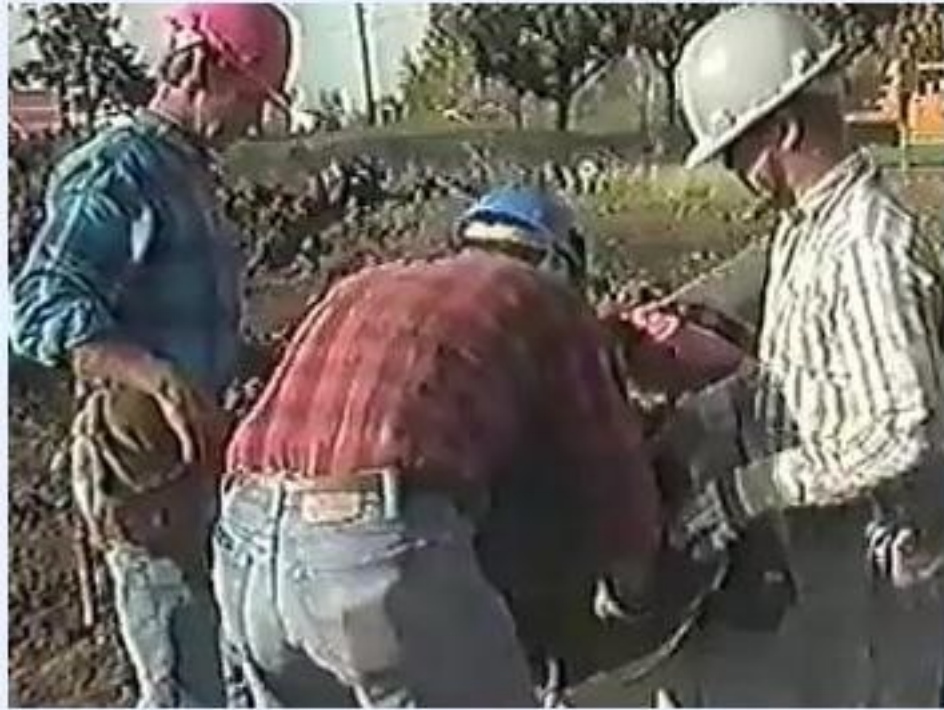
Three workers in hard hats and plaid shirts working together at the entrance of a large pipe, demonstrating teamwork and hazard awareness.
