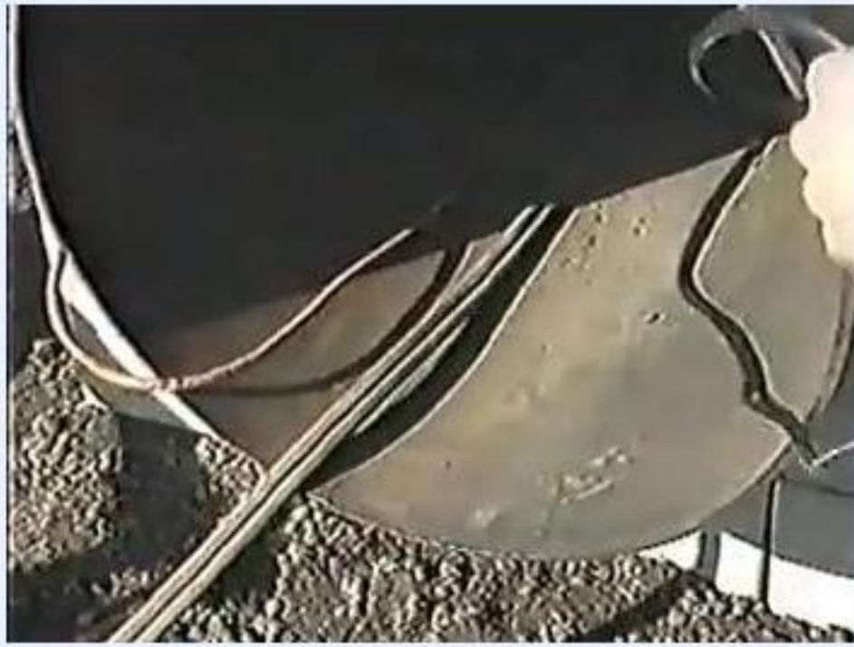
Wide view of the pipe entrance with an oxygen hose trailing inside; the pipe is partially covered with cloth, moments before a fire broke out.
