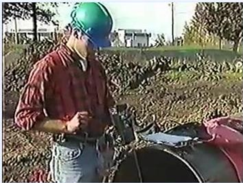
Worker in a green hard hat and gloves placing a wooden board into a large pipe to allow safer confined-space entry.
