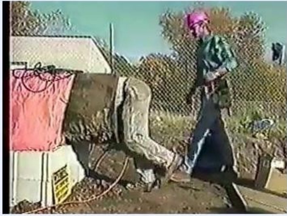
Worker bending over to handle blocks at a construction site, shown within a video frame overlay.
