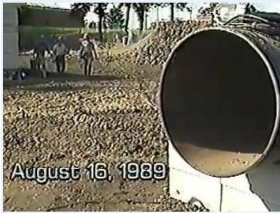
Three workers in hard hats and work attire walking toward a large pipe at a construction site.
