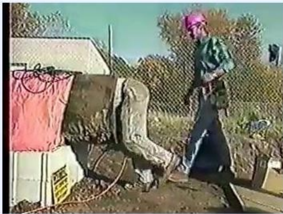
Worker climbing into a pipe while another worker stands by, both wearing hard hats and PPE.
