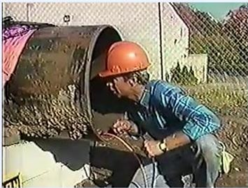
Worker in an orange hard hat crouching near the entrance of a large pipe, speaking into a communication device.
