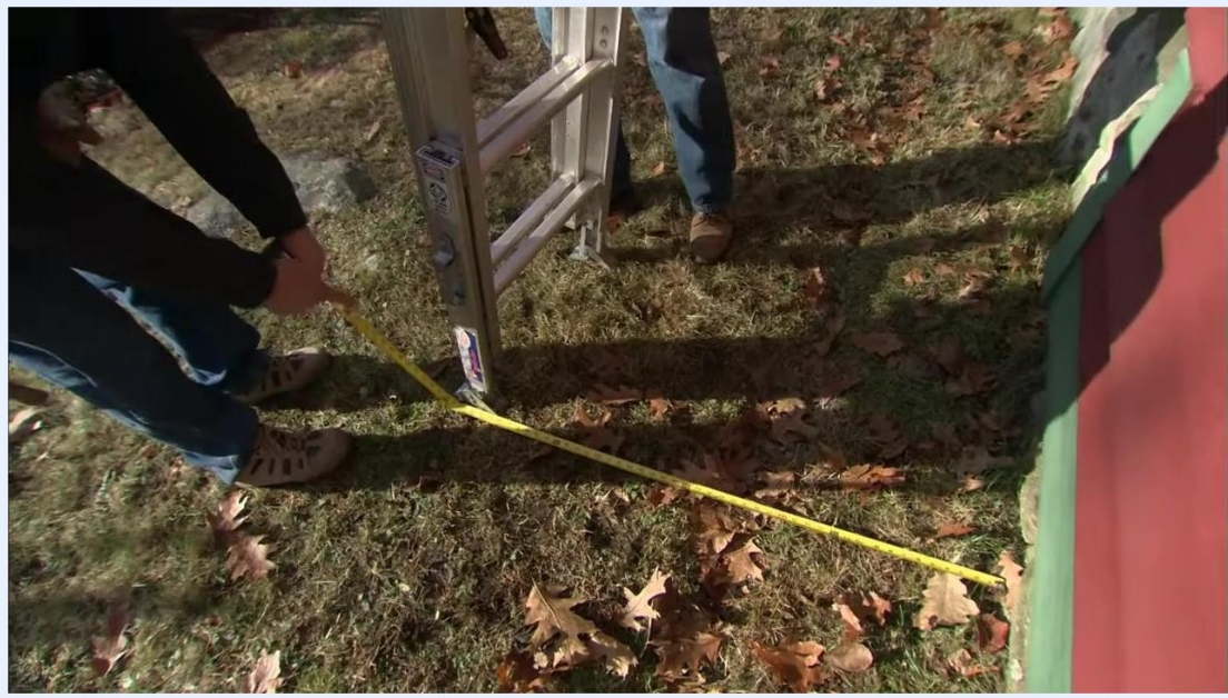
A close-up of a tape measure checking the distance from the base of the ladder to the building, with two people's legs and feet visible.
