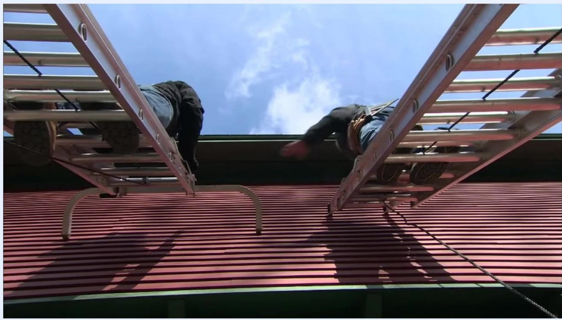
Two extension ladders with stabilizers attached at the top are set against a red building with green roof trim, keeping them clear of the gutter as two people climb.
