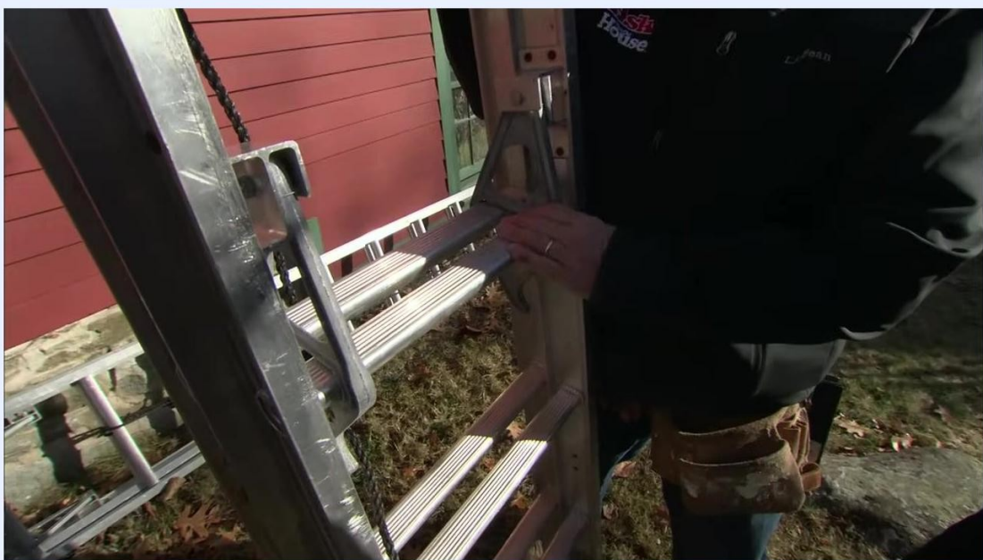
One person lifts and positions an extension ladder upright, angling it toward a building in an outdoor yard.
