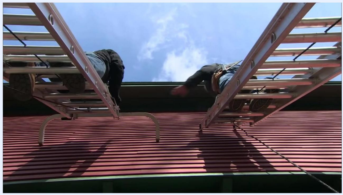
Two people demonstrate the correct side placement of an extension ladder with a stabilizer against a red building.
