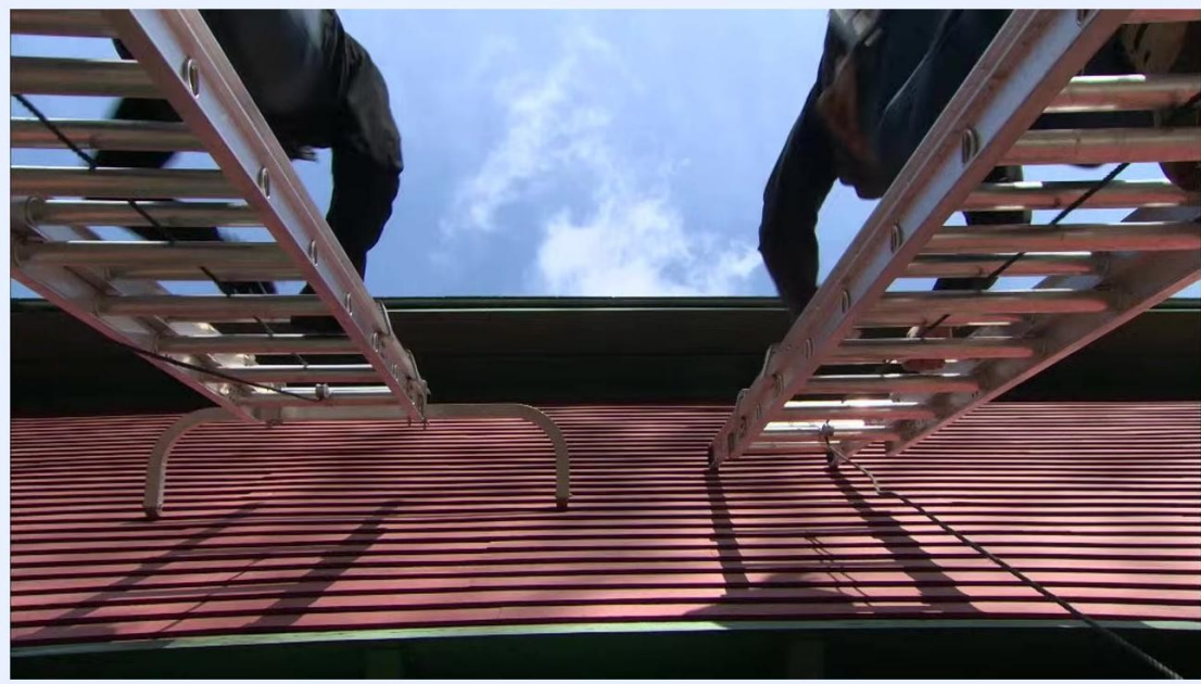
Two ladders with stabilizers attached at the top rest against the edge of a red building's roof, viewed from below as two people climb.
