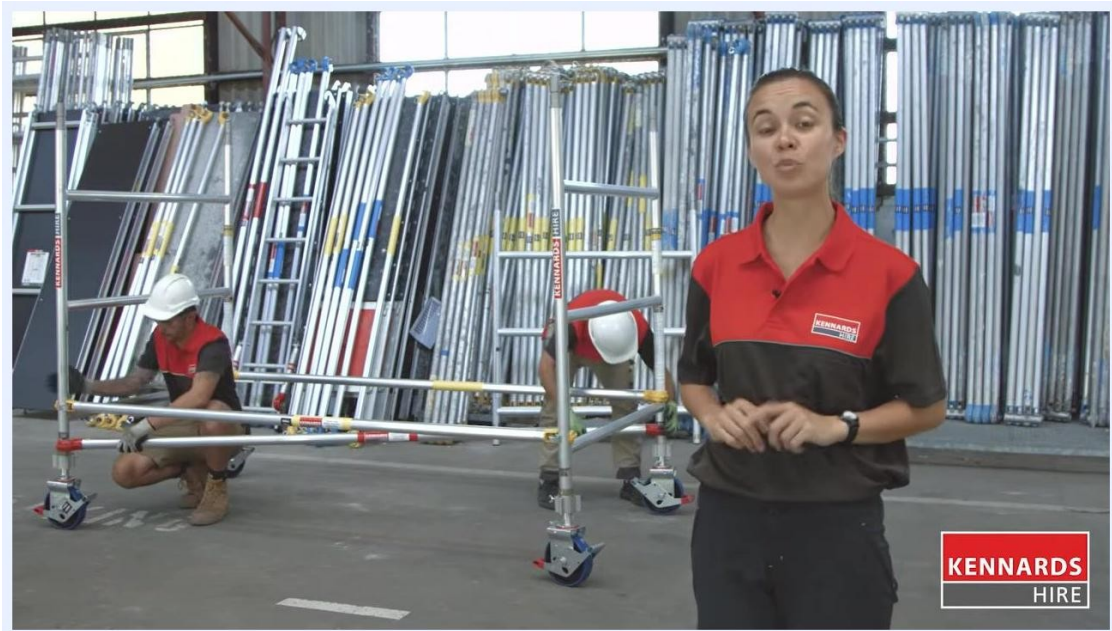
Partially assembled scaffold with the temporary platform installed
