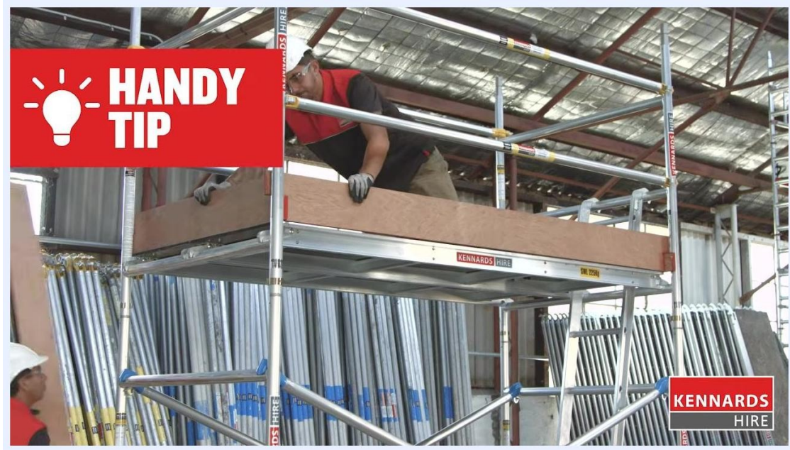
Worker installing the hatch deck on the upper platform, with a handy tip displayed
