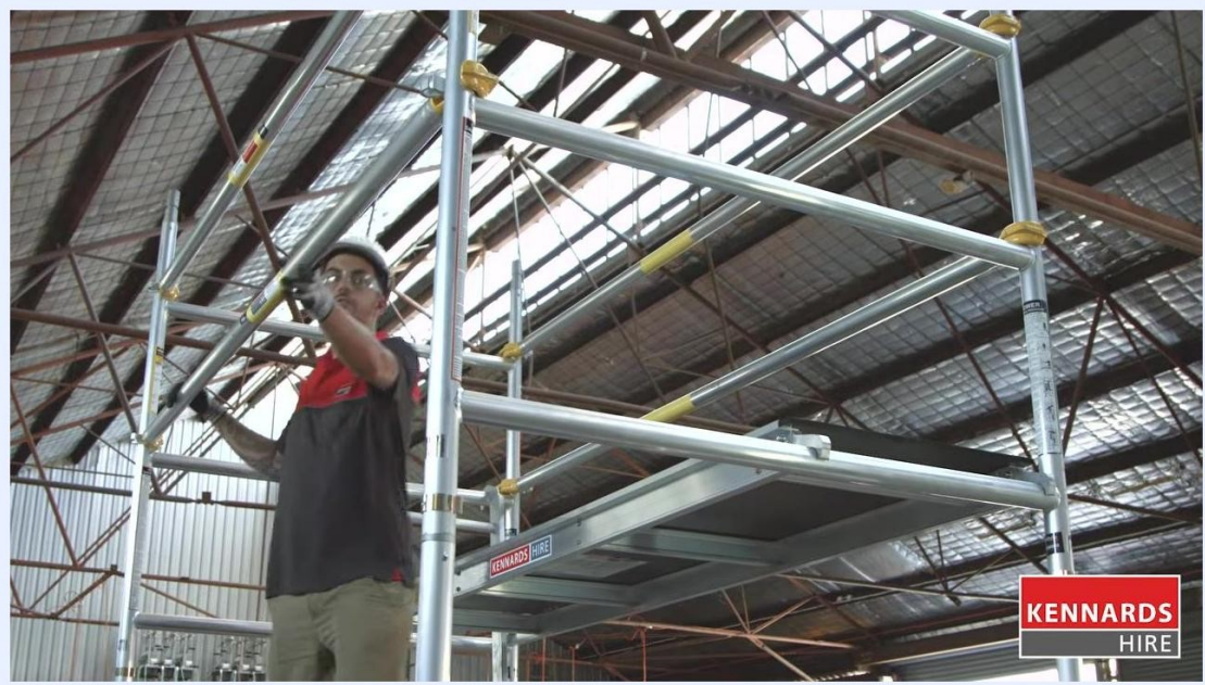
Worker adjusting the platform to align with the working platform height
