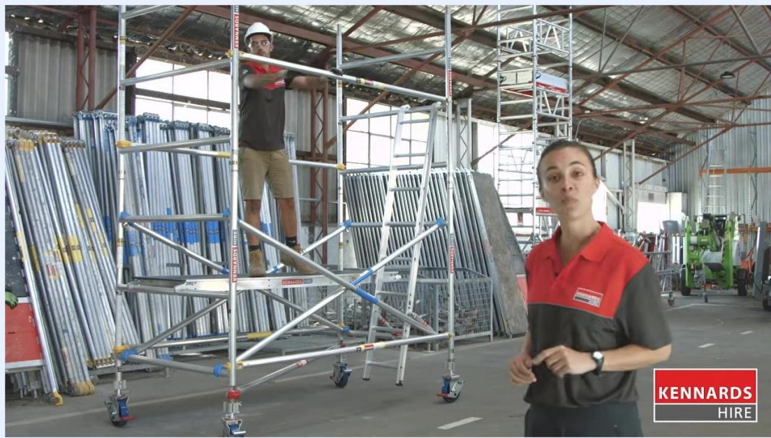
Worker kneeling to secure the ladder inside the scaffold
