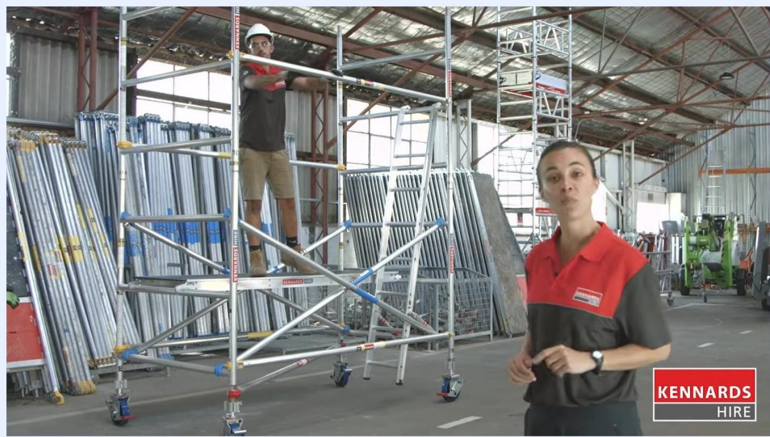
Worker repositioning the hip guard to create a mid rail on the scaffold
