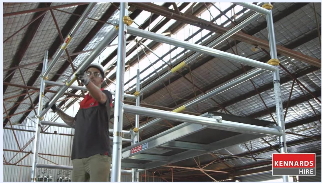
Worker installing an outrigger for additional stability as scaffold height increases
