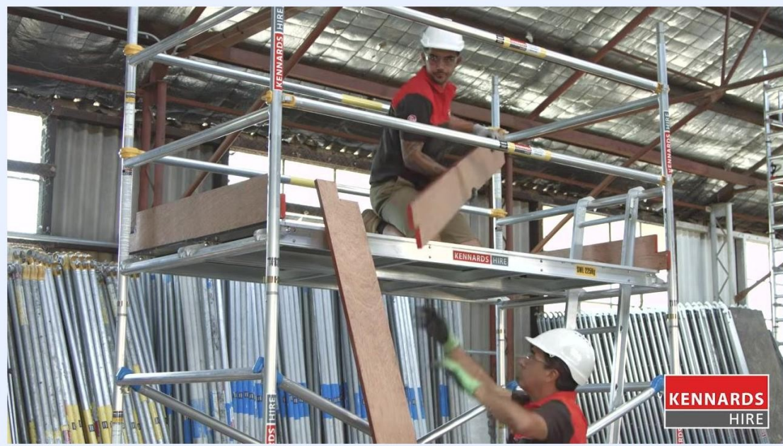
Worker installing wooden toe boards on the upper platform while another worker hands up a board
