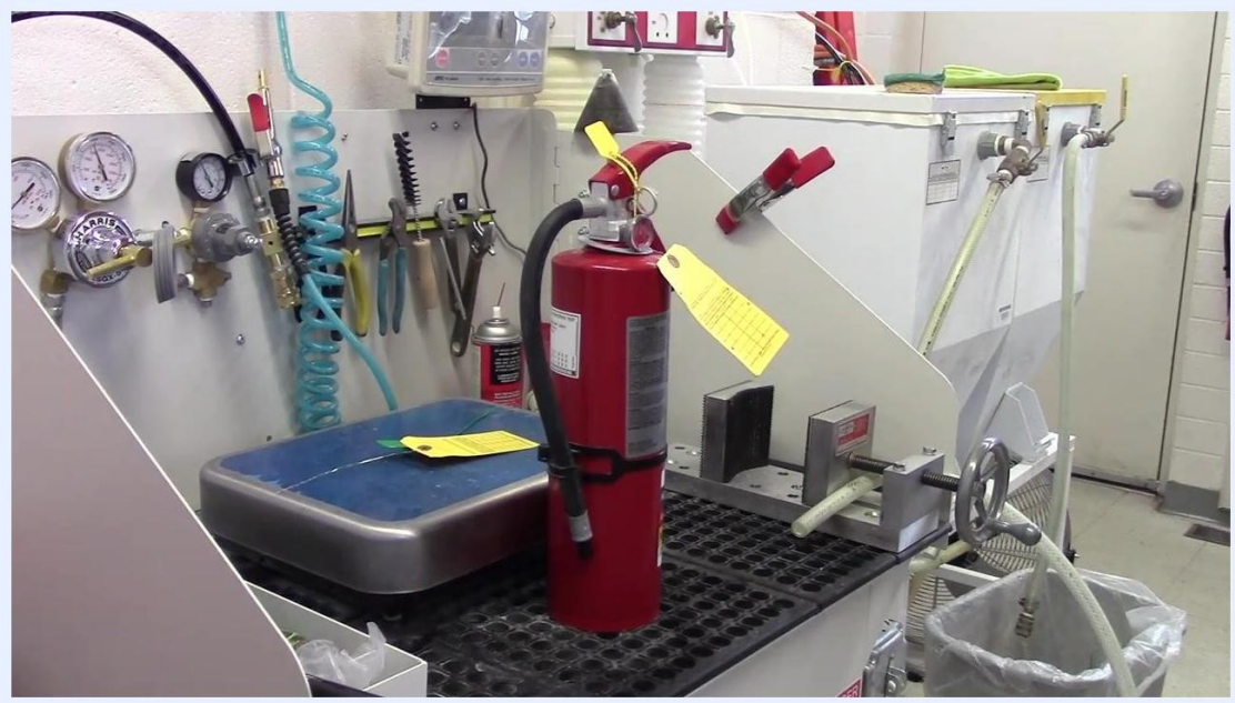
A fire extinguisher placed upright on a workbench in a maintenance area, surrounded by tools, gauges, hoses, and inspection tags.
