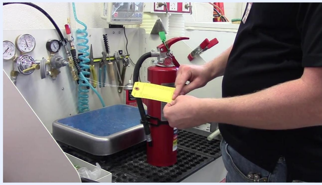
A person holding a new yellow inspection tag, preparing to punch and attach it to the fire extinguisher.
