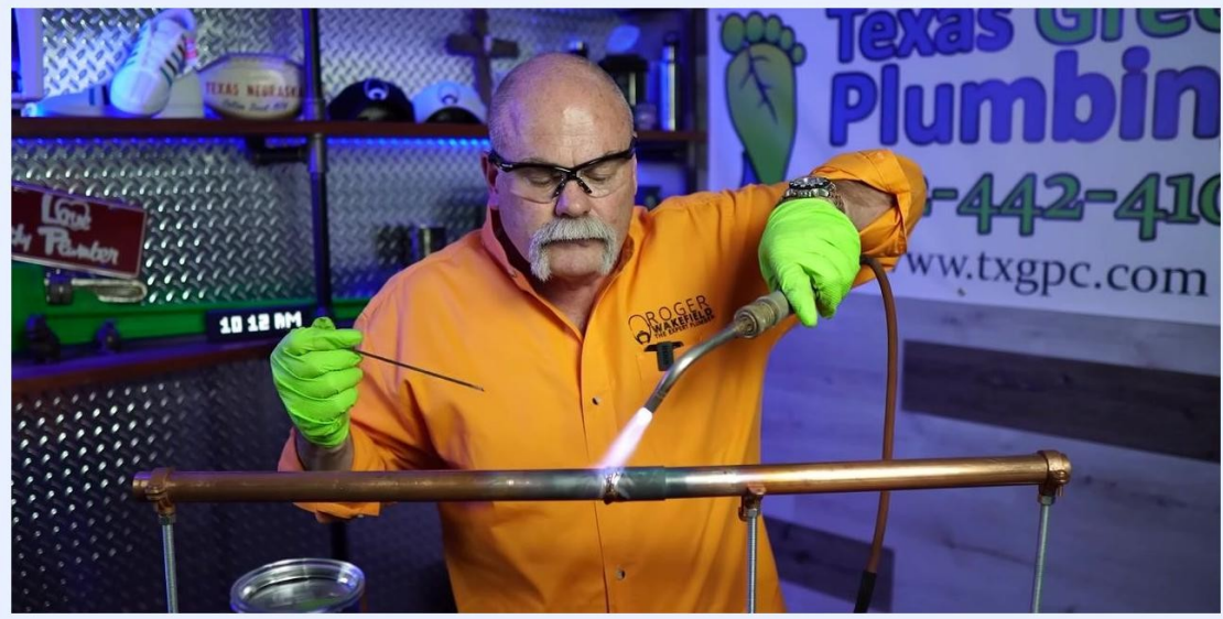
A person continues to heat a copper pipe joint with a torch, closely monitoring the process.
