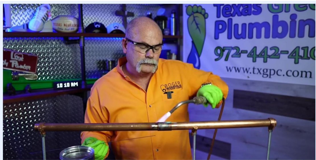
A person alternates between heating a copper pipe joint with a torch and applying solder wire.
