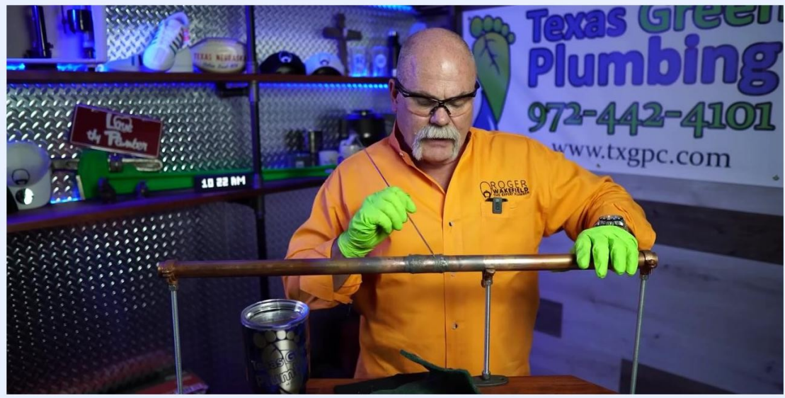
A person uses a flashlight to inspect a cleaned copper pipe joint.
