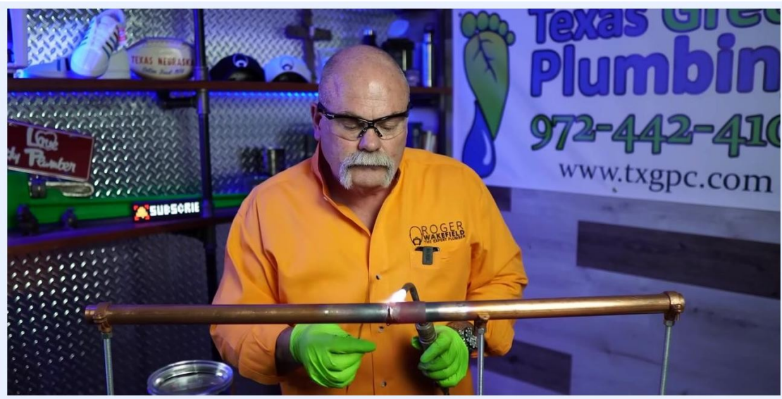
A person performs a final heating pass on a soldered copper pipe joint and inspects the seal.
