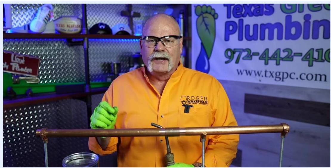
A person holds a plumbing torch below a copper pipe joint, with a flux container placed nearby on the workbench.
