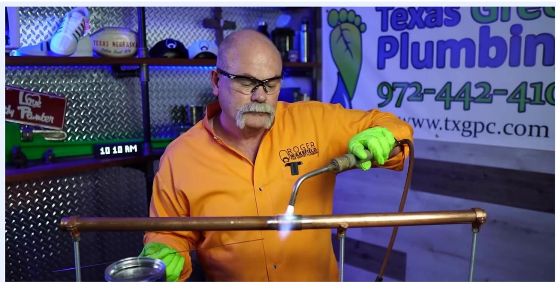
A person continues to heat a copper pipe joint with a torch, ensuring even temperature.
