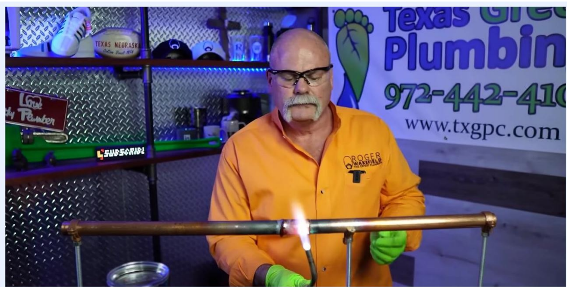
A person stands back, observing a cooling soldered joint with the torch held safely away.
