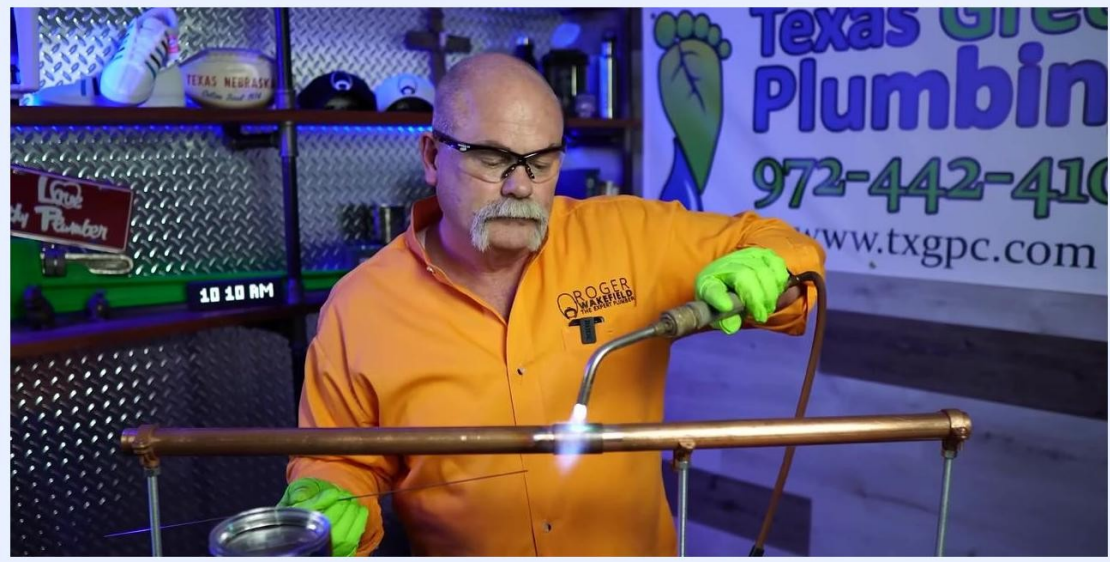
A person applies torch flame directly to a copper pipe joint, heating it for soldering.
