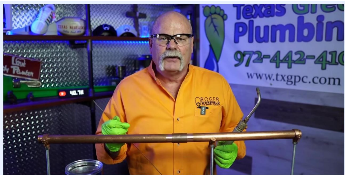
A person holds solder wire and a torch near a copper pipe joint, preparing for the next step.
