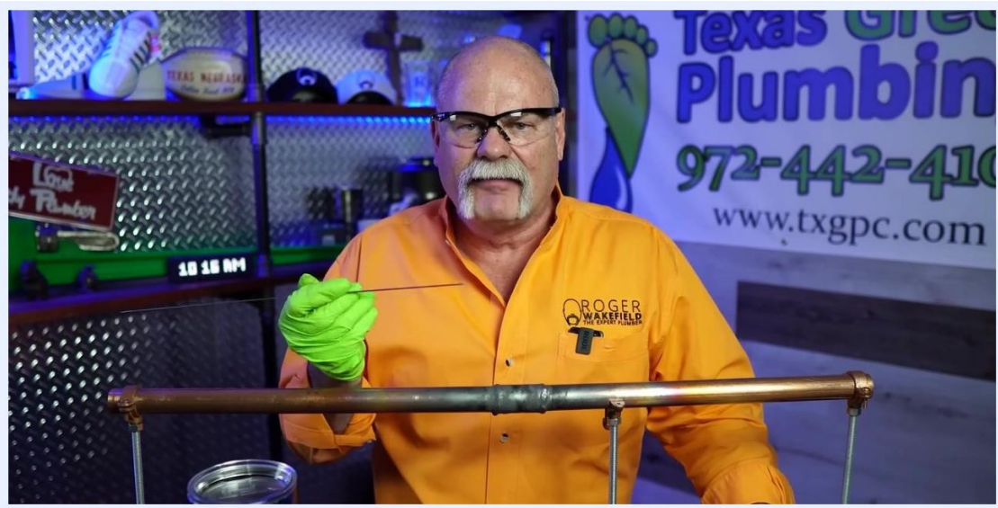
A person presents a completed soldered copper pipe joint, holding up the solder wire for reference.
