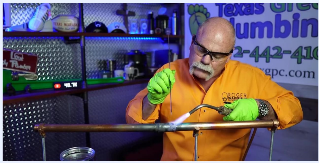
A person finishes soldering a copper pipe joint, holding a torch and solder wire.
