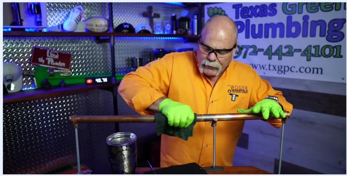
A person uses a green scouring pad to clean a soldered copper pipe joint.
