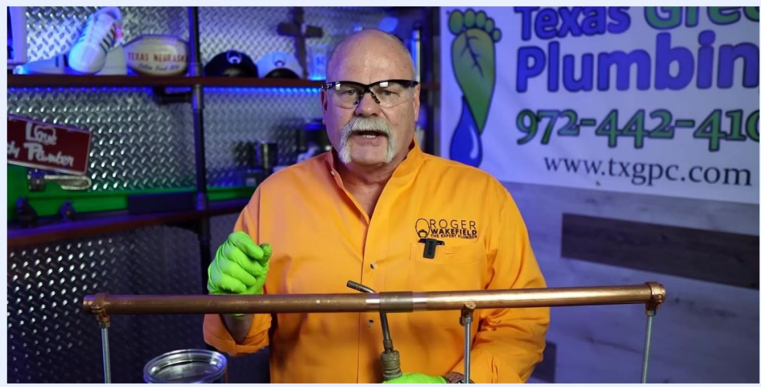
A person holds a torch below a copper pipe joint, applying heat evenly around the connection.
