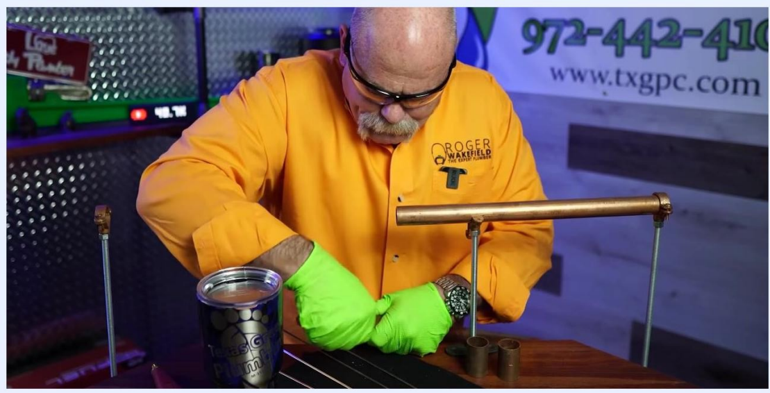
A person wearing an orange shirt and green gloves applies cleaning compound or flux to a copper fitting in a plumbing workshop.
