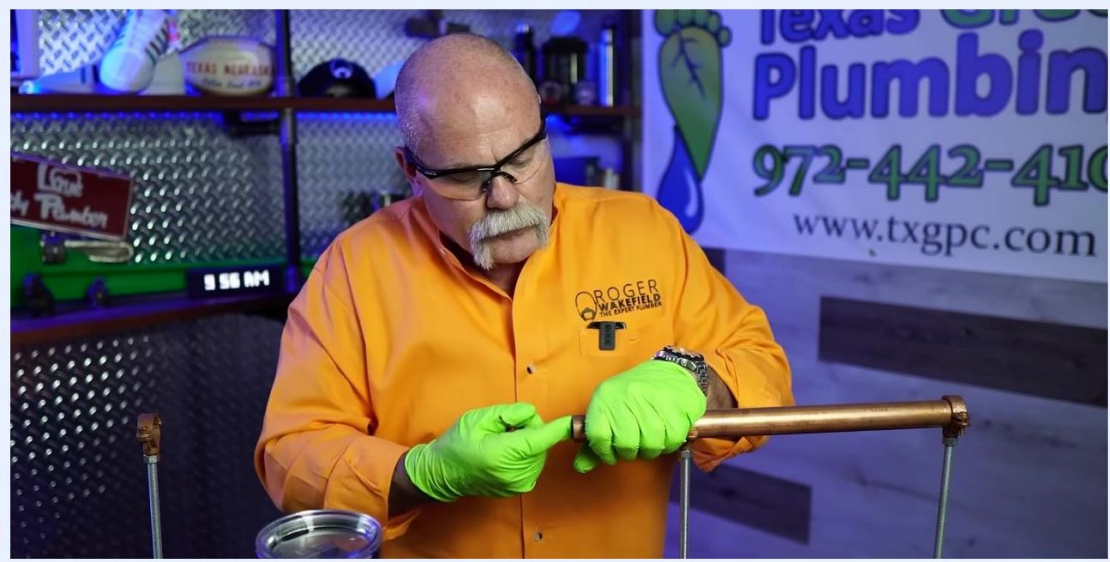
A person wearing safety glasses, green gloves, and an orange shirt uses an abrasive cloth to clean a copper pipe in a plumbing workshop.
