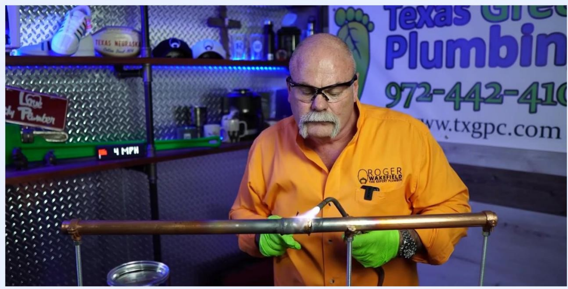
A person applies solder to a heated copper pipe joint with a torch.
