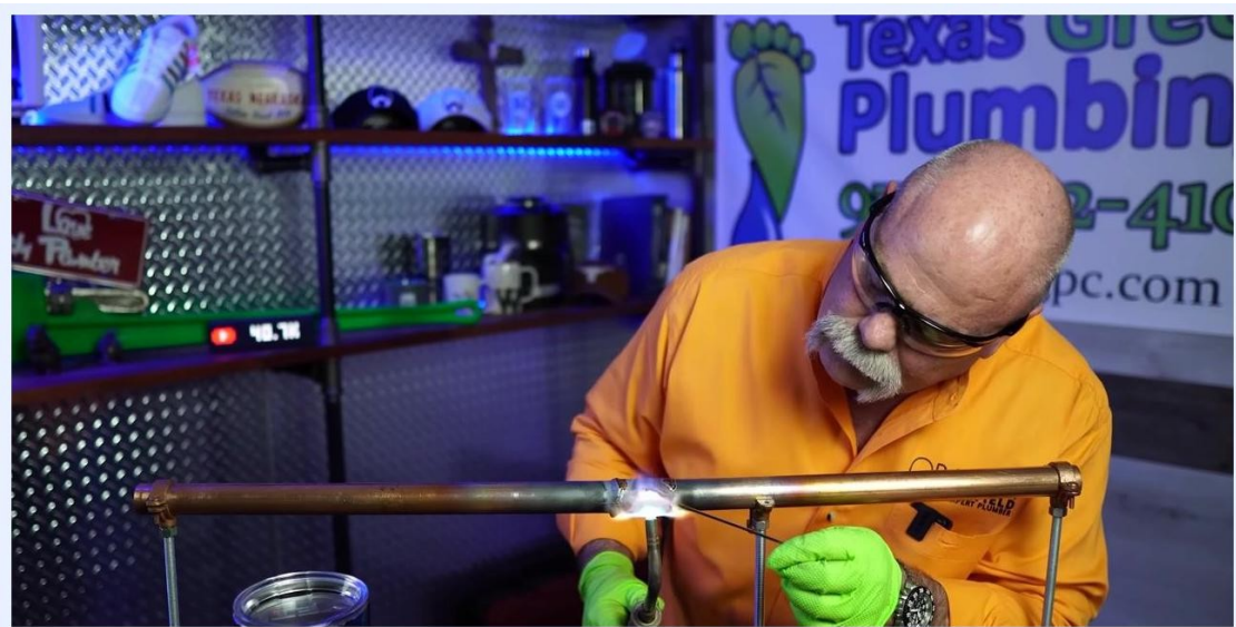
A person applies final heat and solder to a copper pipe joint, ensuring a complete and even seal.
