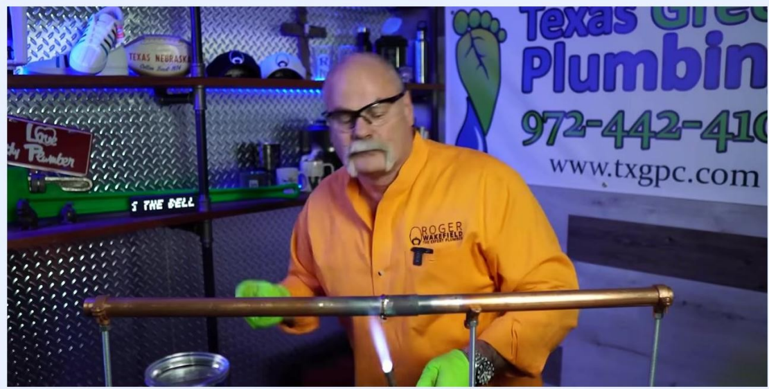
A person removes the torch from a completed soldered copper pipe joint, allowing it to cool.
