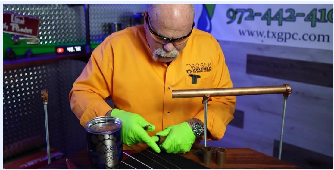
A person wearing an orange shirt and green gloves attaches a copper fitting to the cleaned end of a copper pipe.
