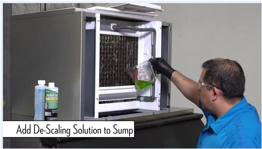
Technician pouring green descaling solution from a measuring cup into the sump.
