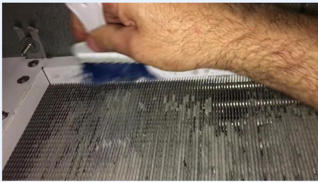
Hand brushing the foamed evaporator coil, with visible cleaner and loosened debris
