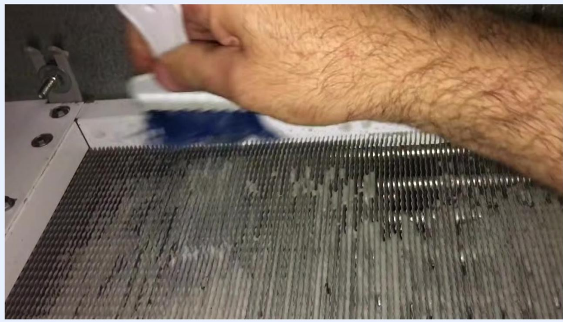
Close-up of evaporator coil fins with foaming cleaner showing texture and buildup being addressed
