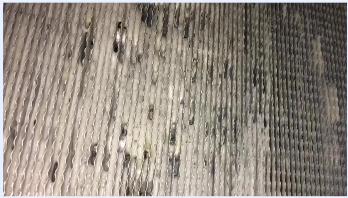
Brass nozzle positioned above the evaporator coil, ready for rinsing with hot water
