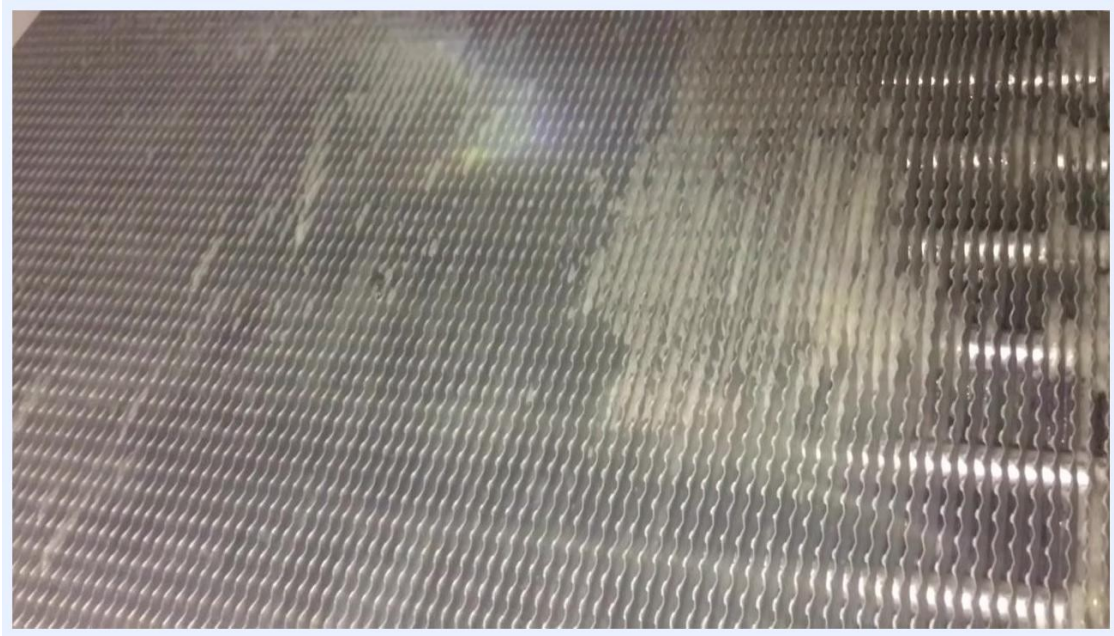
Coil surface with ongoing water spray, showing progress in removing dirt
