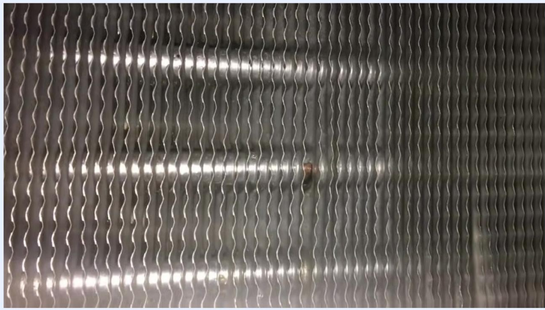
Evaporator unit installed close to the wall, with insulated pipes and food storage containers below
