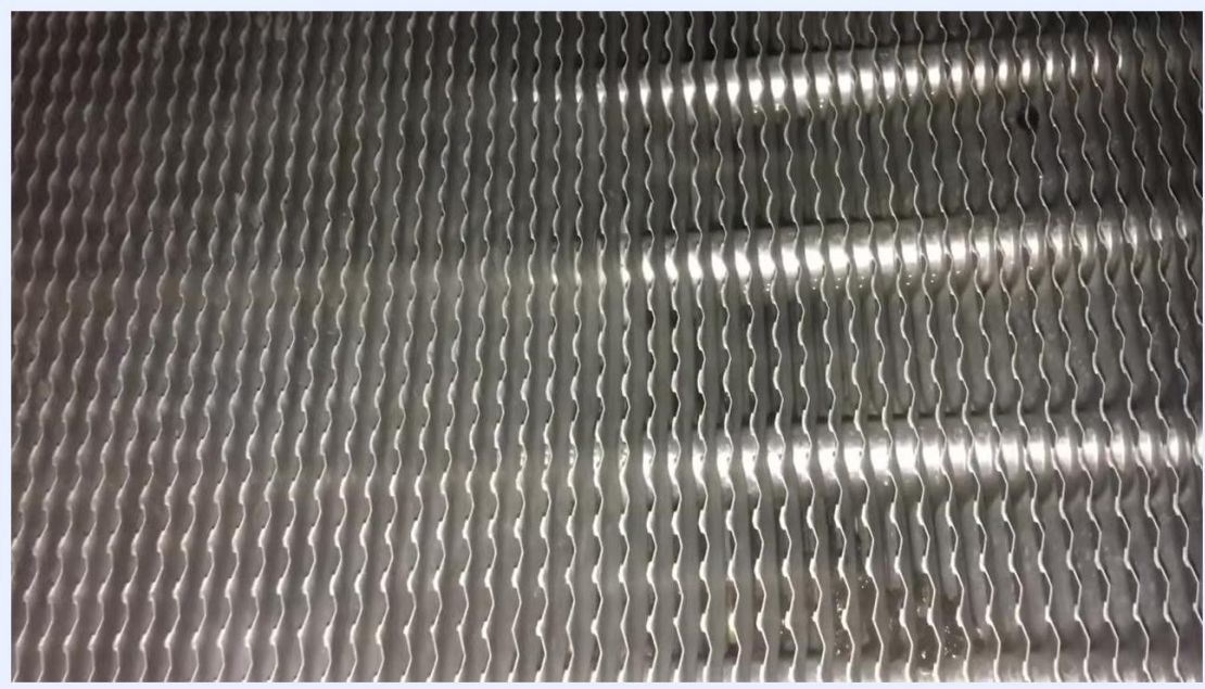
Heat exchanger tubes viewed from a different angle, still clean and metallic
