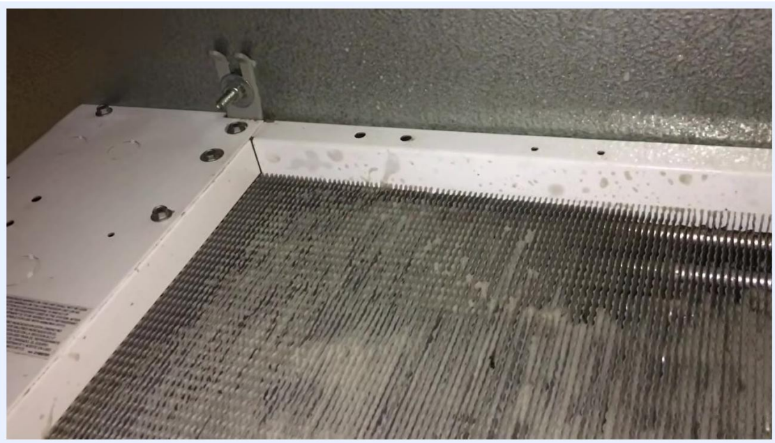
Close-up of coil surface with cleaning in progress and improved cleanliness
