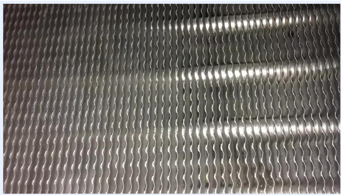
Heat exchanger tubes with a partial view of a white panel and label marking the inspection area
