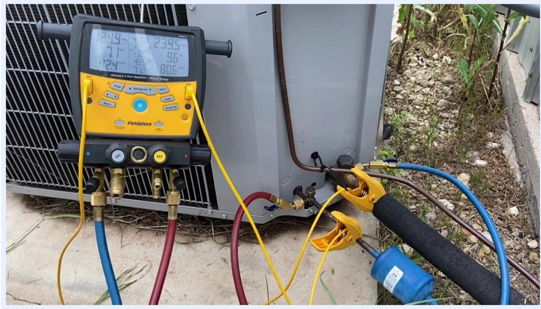
Close-up view of the Fieldpiece gauge display showing the superheat and subcooling values, with hoses and clamps still attached to the AC unit.
