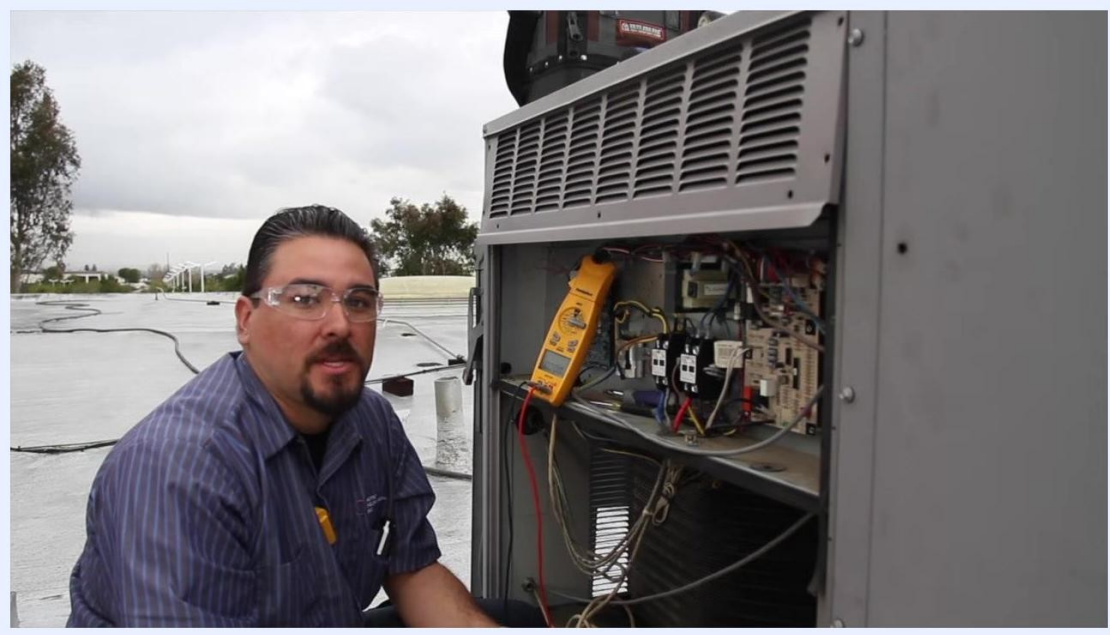
Technician inspecting the blower housing and pulley inside the HVAC unit, checking for wear, alignment, and bearing condition.
