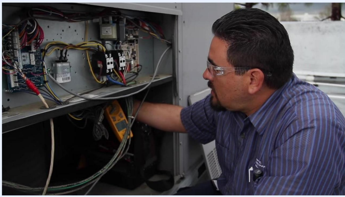
Technician measuring supply vent temperature at the labeled panel of the HVAC unit.
