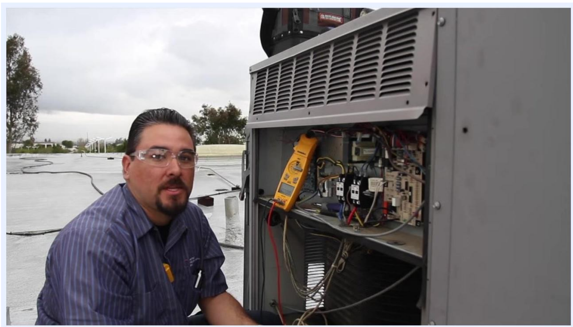
Technician using a multimeter set to microfarads to test the capacitor inside the open electrical compartment.
