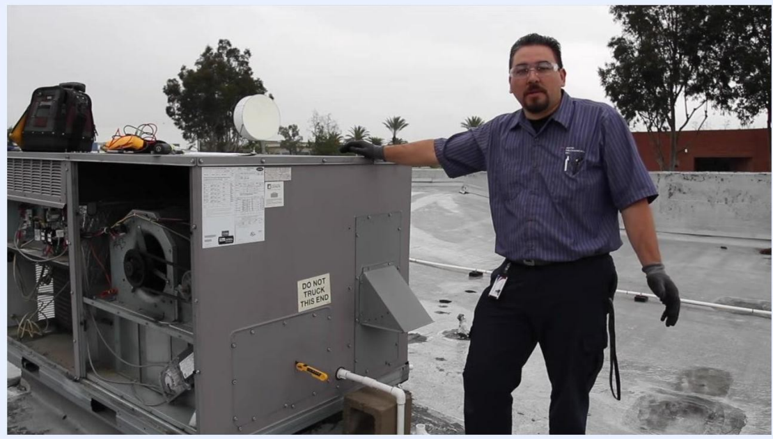
Technician holding the drive belt and preparing to reinstall it onto the blower pulley, with the pulley and belt path clearly visible.
