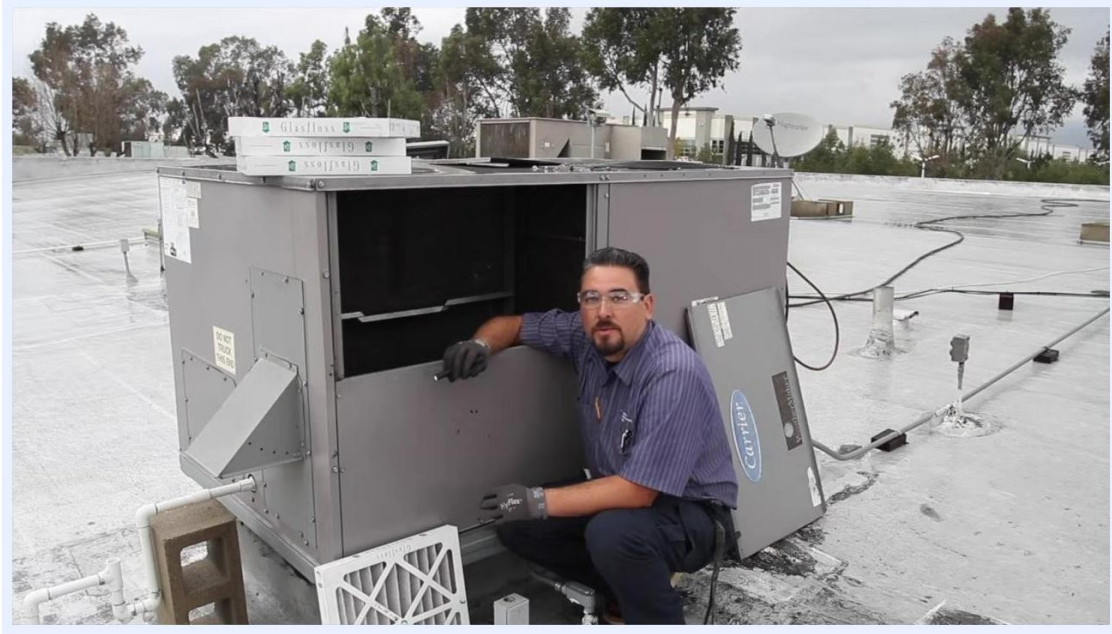
Technician at the HVAC unit, preparing to clear the drain lines.
