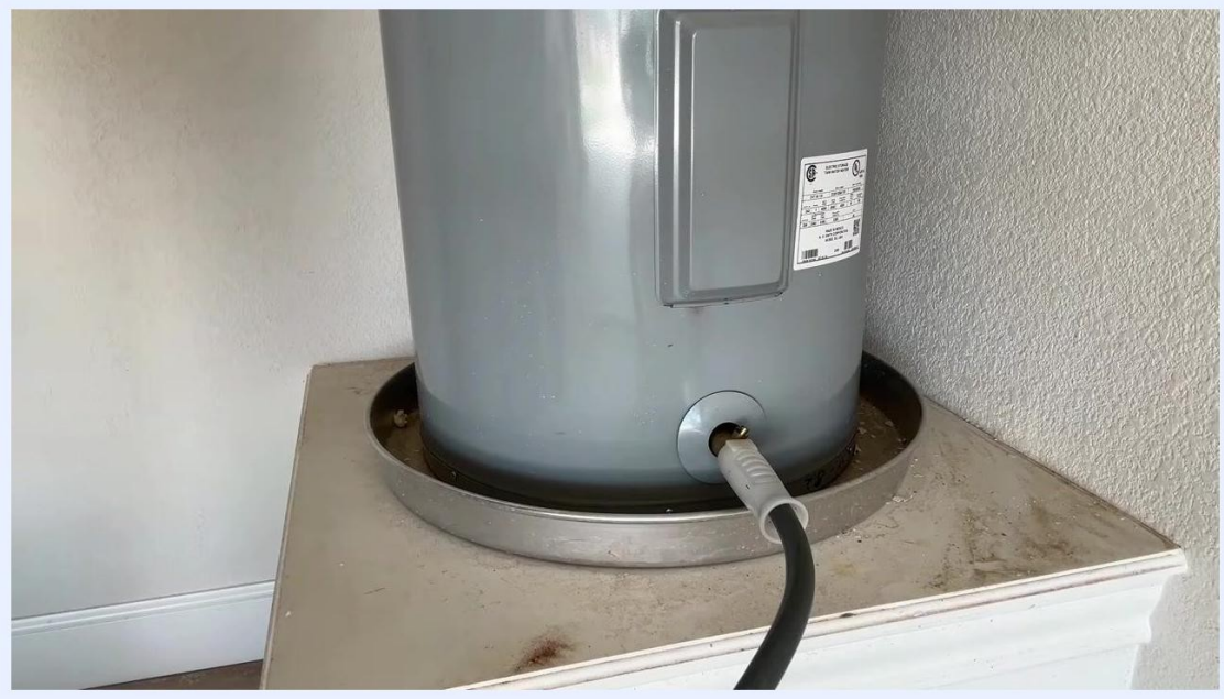
Person explaining the draining process next to the water heater, with hose attached and water draining.
