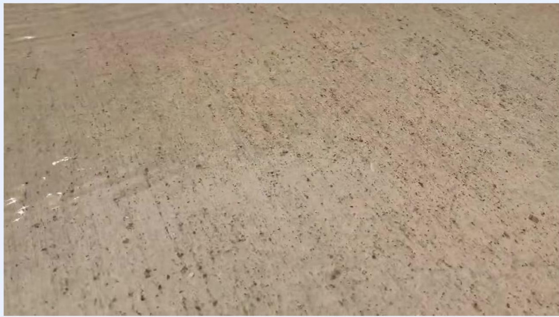
Concrete surface with scattered dark sediment particles and a thin layer of water, showing sediment flushed from the water heater
