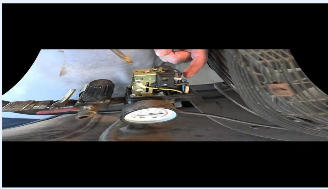
Hand using a screwdriver to adjust the top screw on the pressure switch, with the pressure gauge and wiring visible
