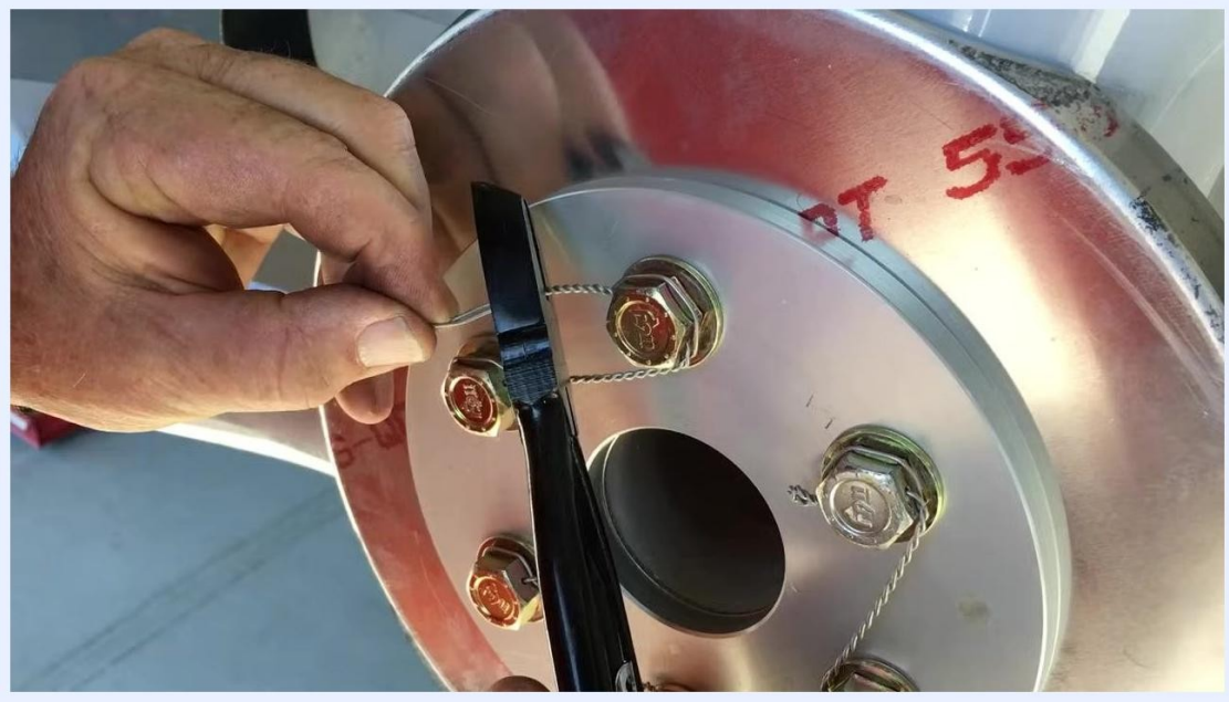
Hand-twisting the tag end (pigtail) of the safety wire in the opposite direction, using pliers for precision, with the wire aligned to the bolt hole
