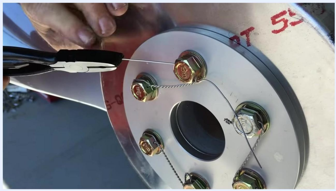
Completed section of safety wire with tag end positioned, bolts secured, and wire tightly twisted
